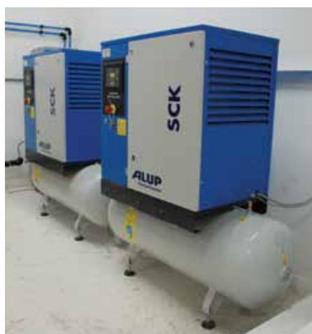
Two compressors on buffer vessels
